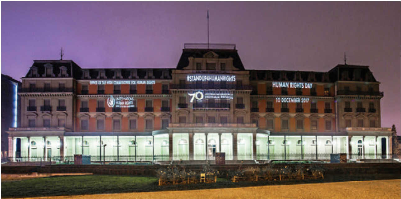
The façade of Palais Wilson, UN Human Rights headquarters in Geneva, illuminated on Human Rights Day, December 2017. © OHCHR
